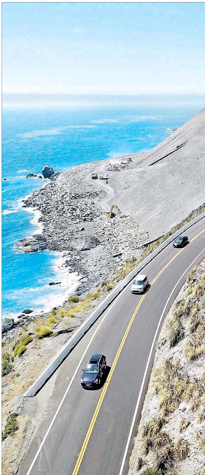
VEHICLES ZIP along the newly reconstructed California 1 roadway in early August, site of last year's Mt
